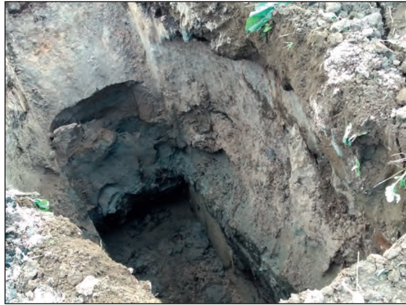
Test pit 5a, looking south east
