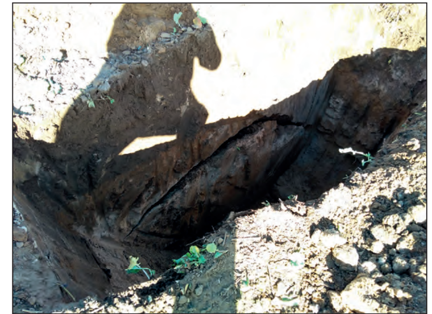
Test pit 11, looking north west
