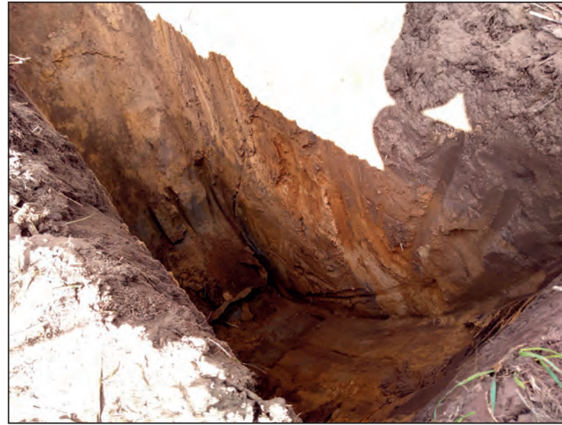
Test pit 6, looking north
