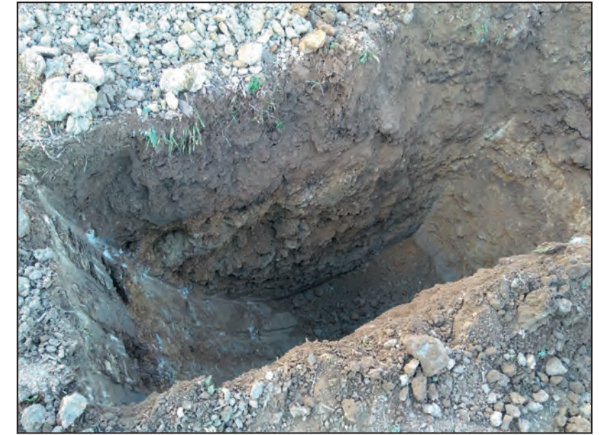
Test pit 7, looking south
